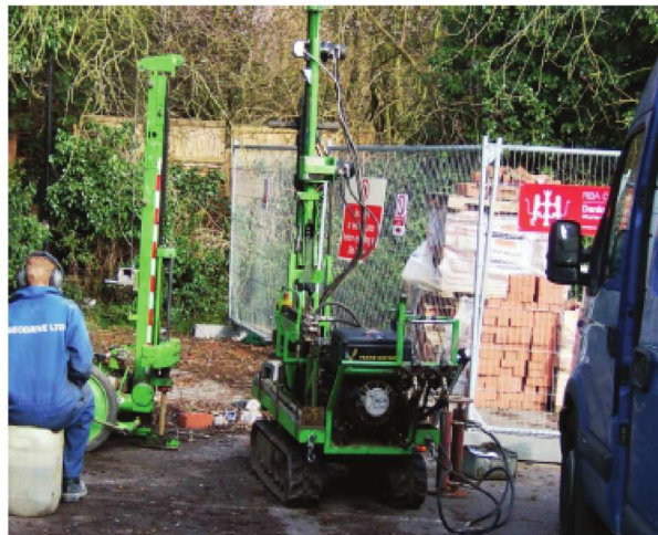
Figure C.16 — Small percussion (RHS) and SPT rigs (LHS)
