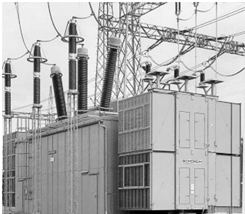
Figure B.3 — Outdoor transformer in enclosure
