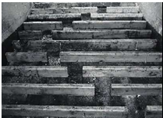
a) Baffles installed on a weir shown under dry conditions
