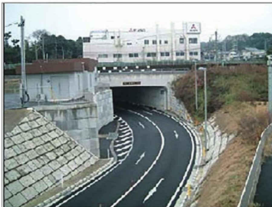
Figure D.8 — Flooding condition warning on an underpass
