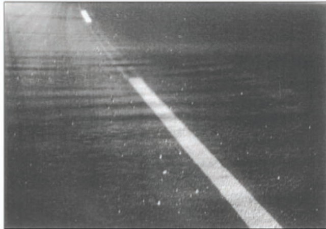
Figure C.9 — Megatexture caused by functioning of finisher
