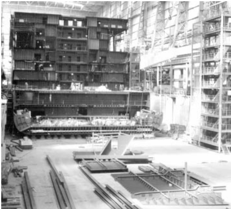
Figure 17 — Bulkheads and decks
