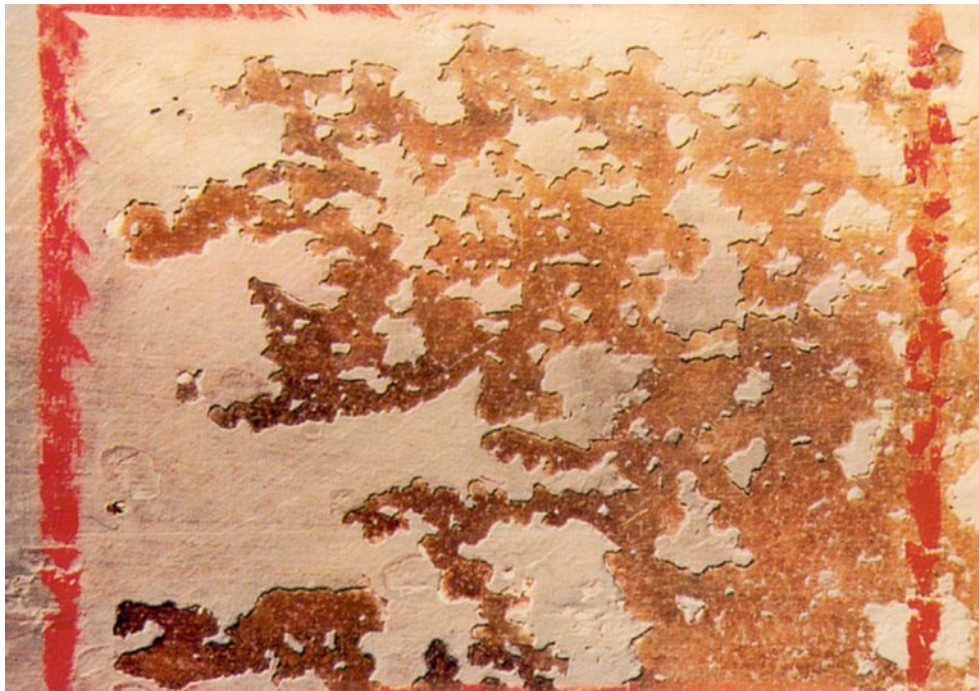
b) section from Figure 12 a): clear illustration of the defect at increased magnification
