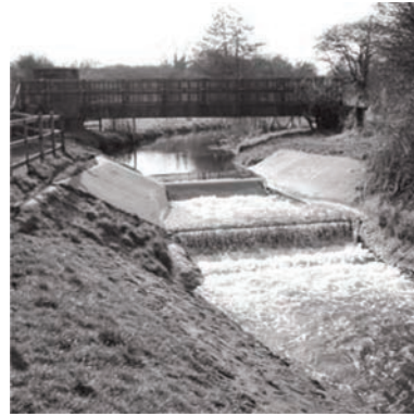
b) Trapezoidal-throated flume
