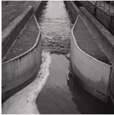
a) Rectangular-throated flume
