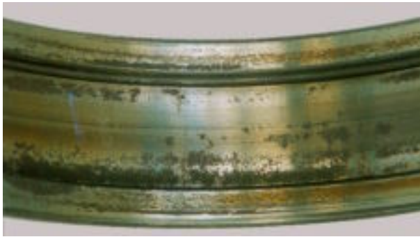
Figure 22 — Corrosion on roller bearing outer ring
