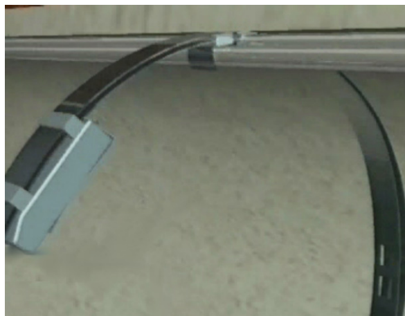
Figure 17 – Spring loaded stainless-steel ring – Conduit fastening
