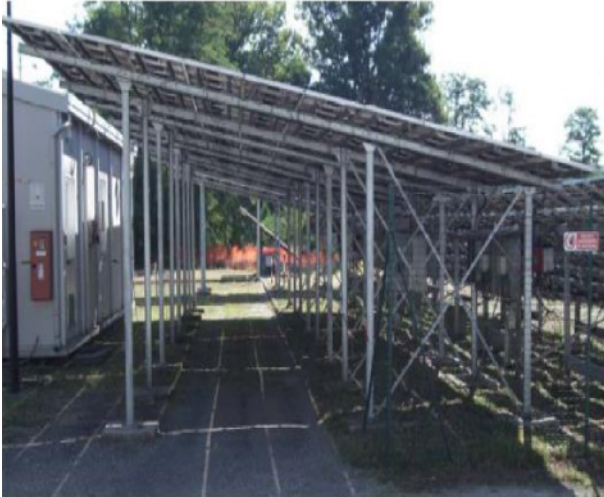
Figure 15 — Photovoltaic panels feeding a single phase inverter directly connected to an LV power line
