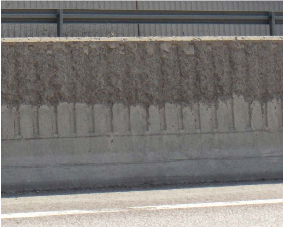
Figure A.2 — Precast concrete element exposed for 5 years to de-icing agent in a highway roadside in Finland
