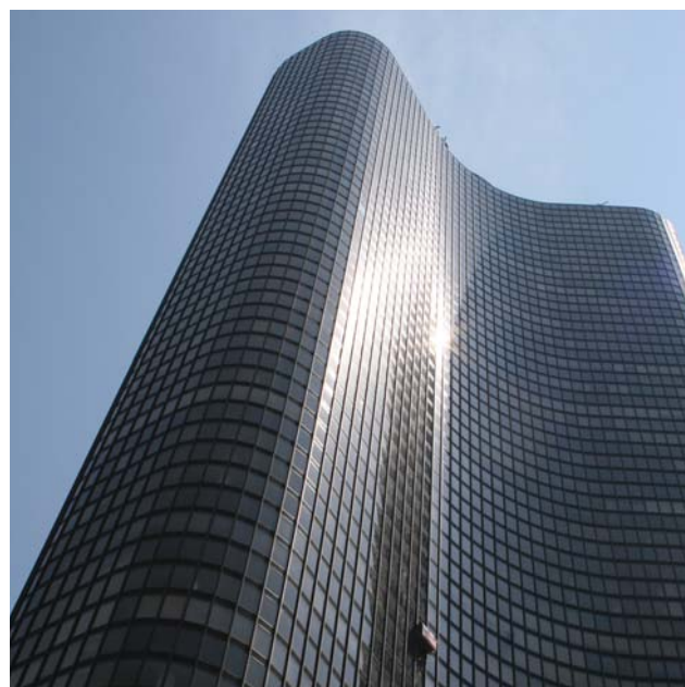
Complex or unusual building arrangements may point towards a performance based design basis.
