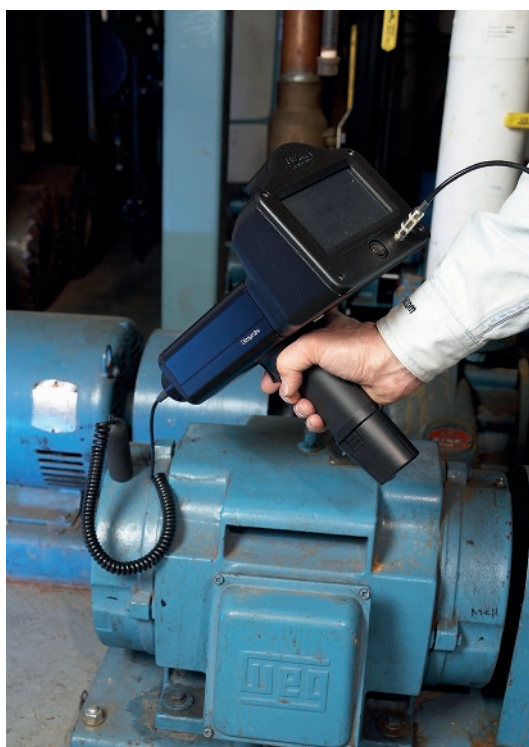
Figure 2 — Example of structure-borne ultrasound monitoring
