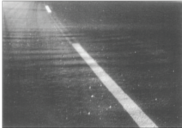
Figure C.9 — Megatexture caused by functioning of finisher
