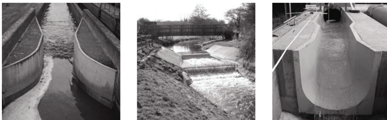
a) Rectangular-throated flume b) Trapezoidal-throated flume c) U-throated flume
