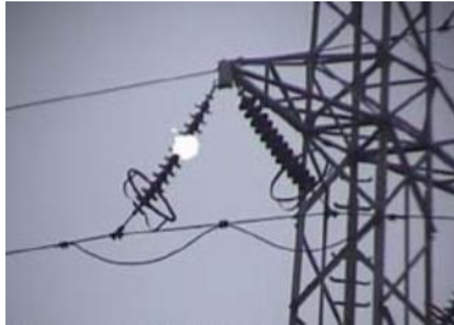
Figure A.28 – Failing external insulation –Example 1
