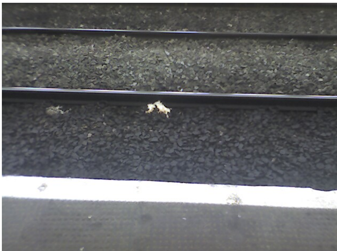
Figure I.1 – Example of ballast covering sleepers
