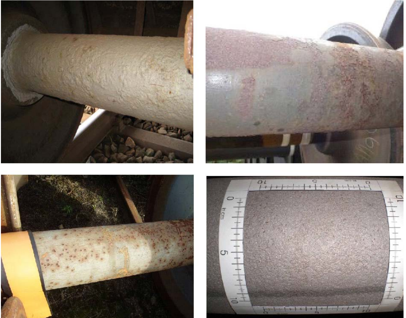
Figure I.2 — Large heavily corroded and uniformly pitted areas
