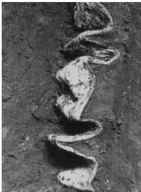
Figure A.5 — Buckling and kinking of drain due to very large relative compression of peat
