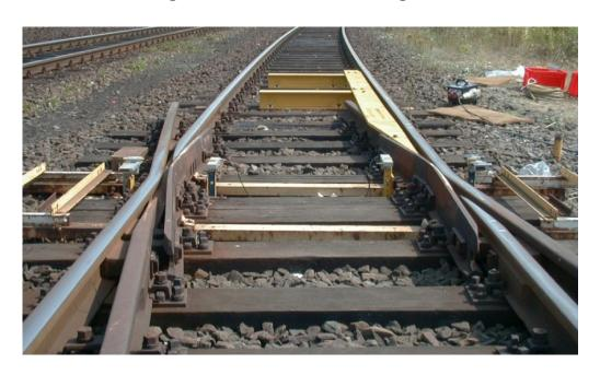
Figure E.3 — Example for curved crossing (DB Systemtechnik, Minden)
