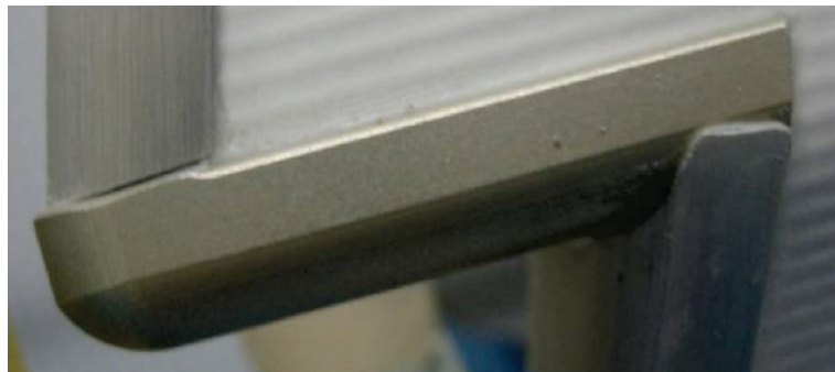
Figure A.16 — Example of an alignment finding
