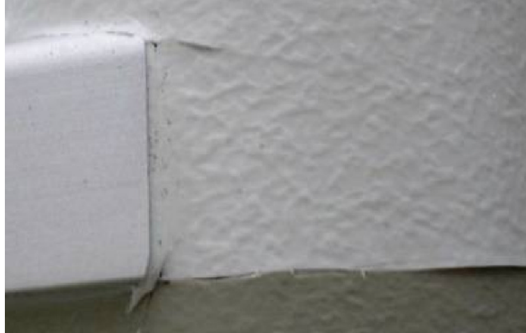
Figure A.12 — Example of poor fit split line finding
