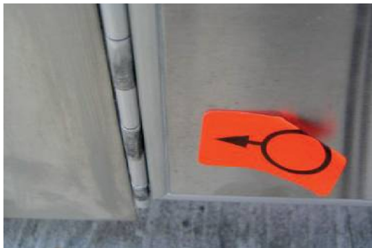
Figure A.21 — Example of a chafing finding
