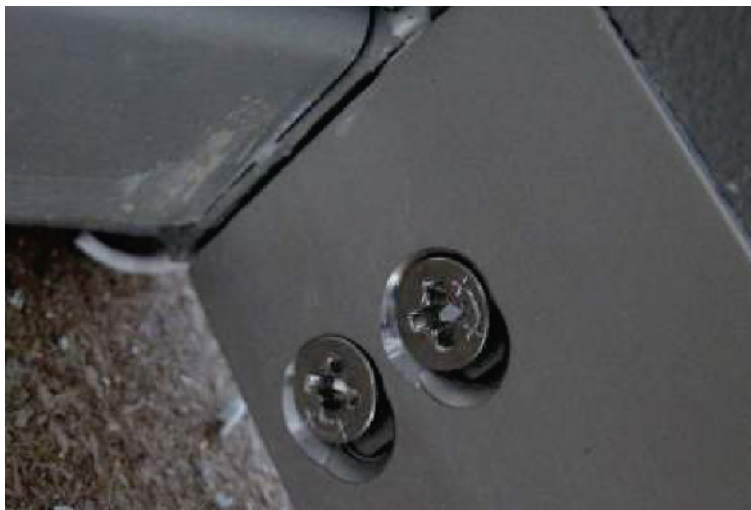
Figure A.33 — Example of a bad hole finding
