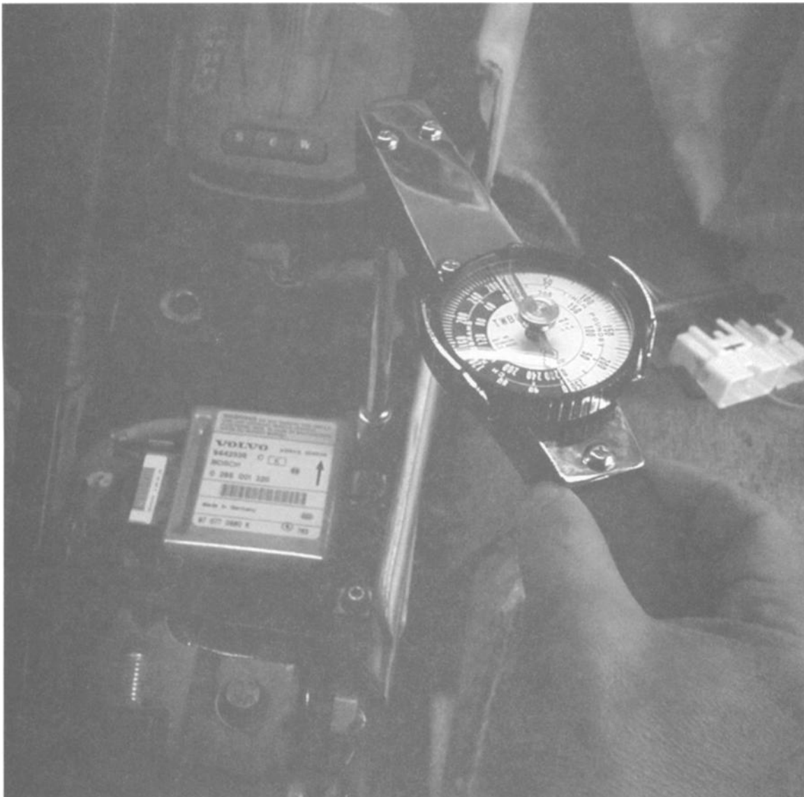
FIG. 5.3—Checking attaching bolt-tightening torques before SRS ECU removal.
