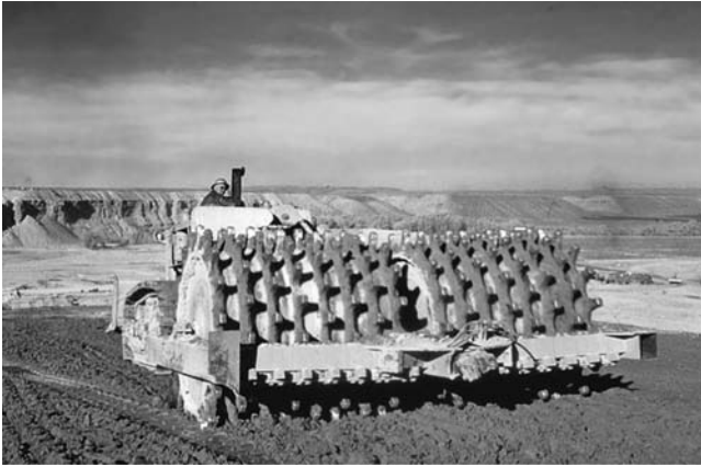
Fig. 1C —Traditional sheepfoot roller—provides a kneading action for plastic soils.
