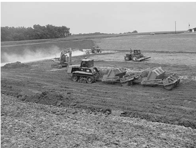
Fig. 3—Linear construction of an agricultural-waste holding pond with a soil amendment.
