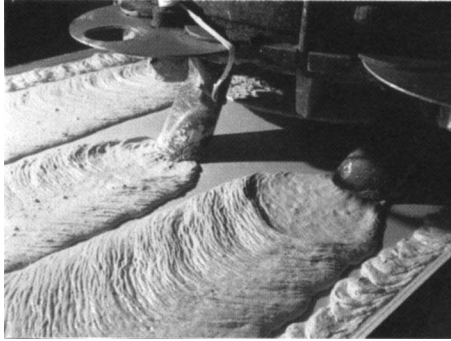
Fig. 7.5 —Three-port mixer depositing slurry onto back of face paper. Note: slurries from edge mixers.
