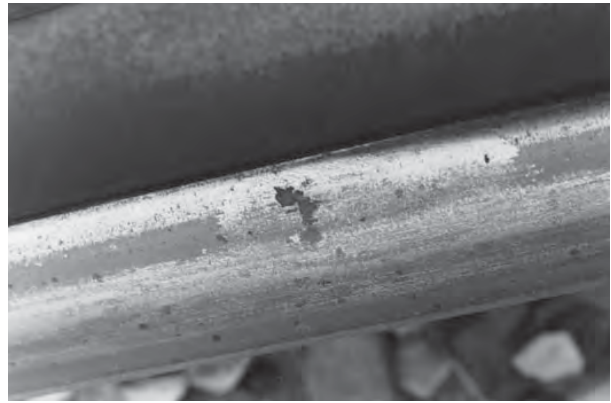
Fig. 9-11—Surface fatigue of railroad track.
