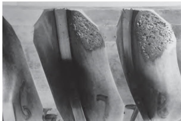
Fig. 9-20—Pitted and spalled worm wheel.
