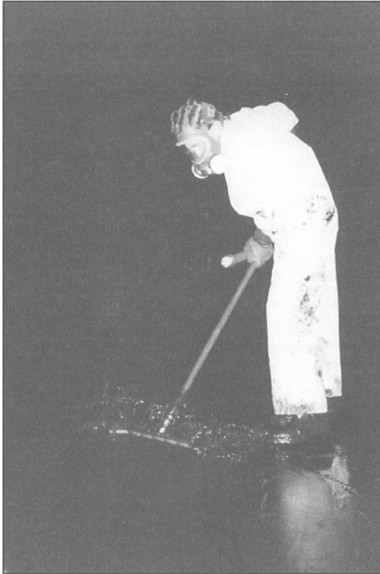
FIG. 1—Bulk storage tank cleaning. Confined space entry certified technician, using squeegee to clean sludge off bottom of terminal tank (high sulfur diesel). Photo courtesy of Fuel Quality Services, Inc.
