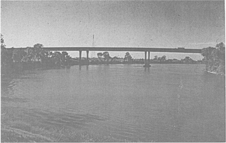
FIG. 15.1 Overall view of Bryte Bend Bridge.
