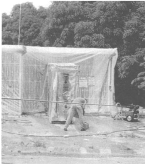
Figure 10.5 Containment for an exterior lead abatement project
