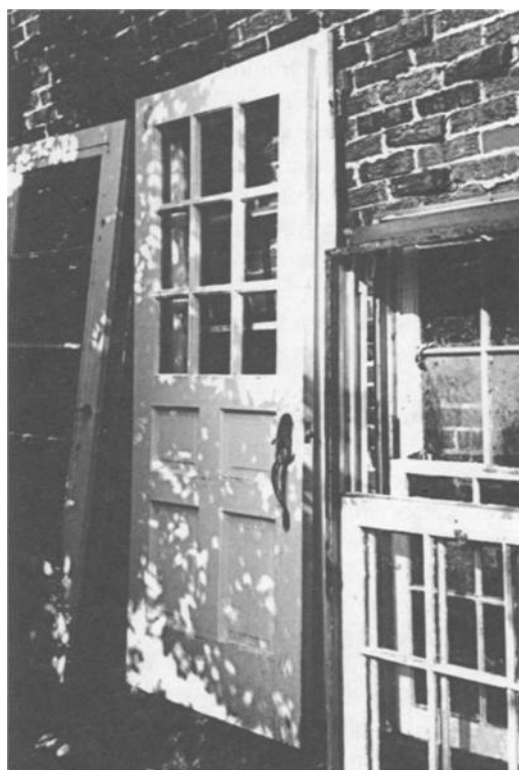
Figure 11.4: Removal and replacement of lead-based paint coated doors and windows
