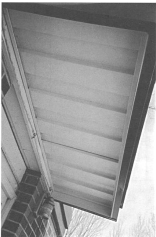
Figure 11.3: Soffit after metal enclosure applied
