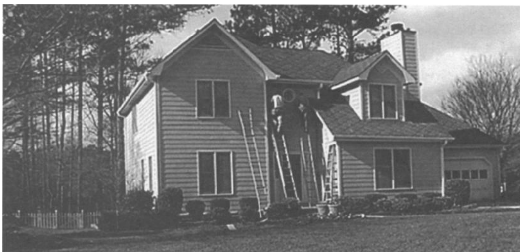
Figure 11.5: Lead hazard control projects are frequently coordinated with renovation activities
