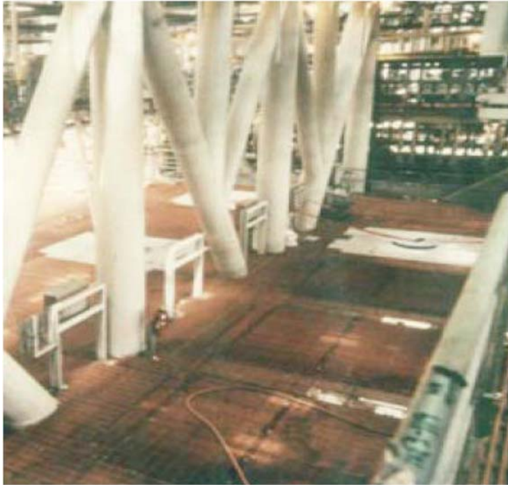
FIG. X1.5 Examples of FRP Gratings Used Offshore: Well-Bay Flooring
