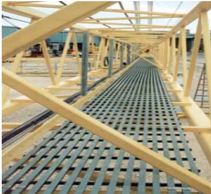
FIG. X1.4 Examples of FRP Gratings Used Offshore: Cranes
