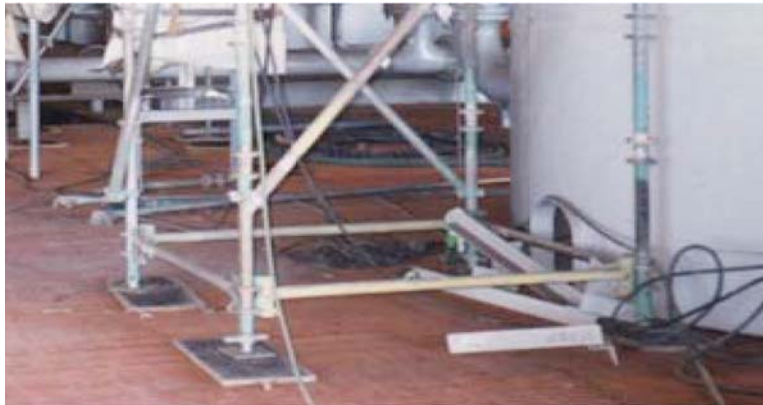
FIG. X1.15 Correct Distribution of Load on FRP Gratings
