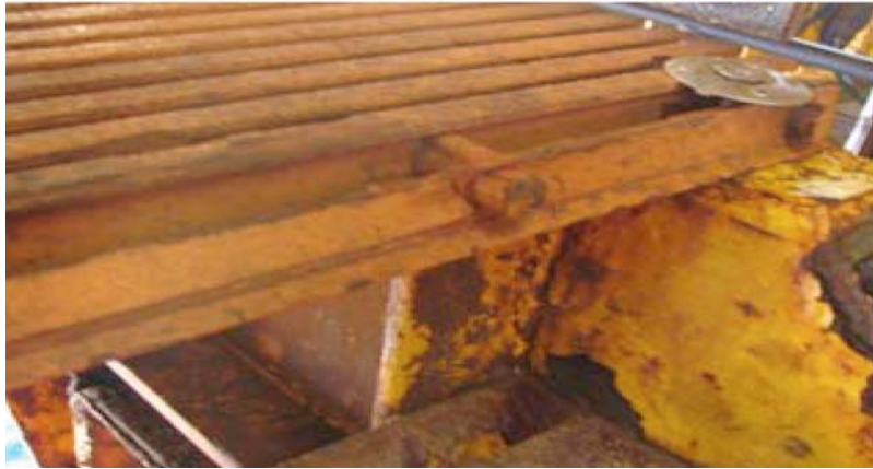
FIG. X1.7 FRP Grating—No Nosing Bar
