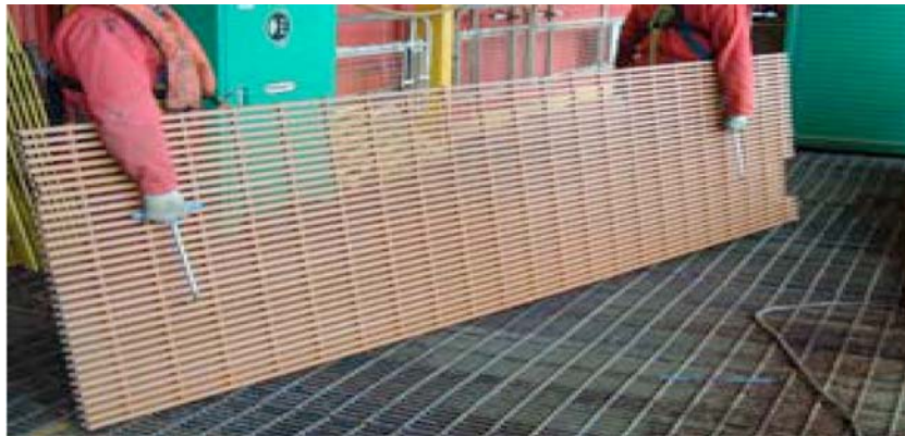
FIG. X1.14 Correct Handling of FRP Gratings
