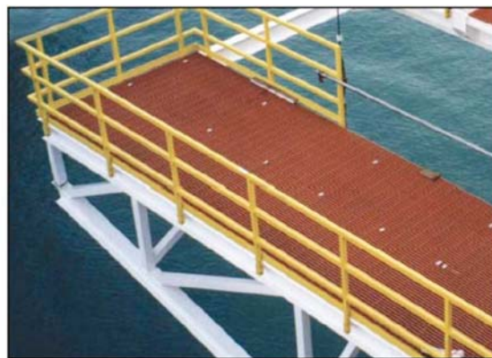
FIG. X1.1 Grating Floor Systems as Used Offshore
