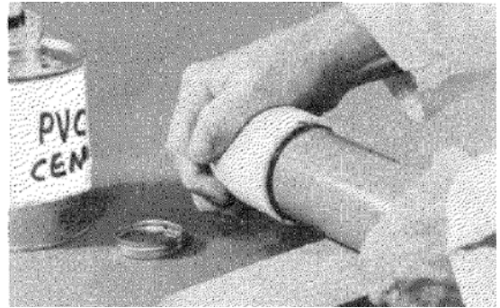
FIG. X3.4 Assembly of Joint
