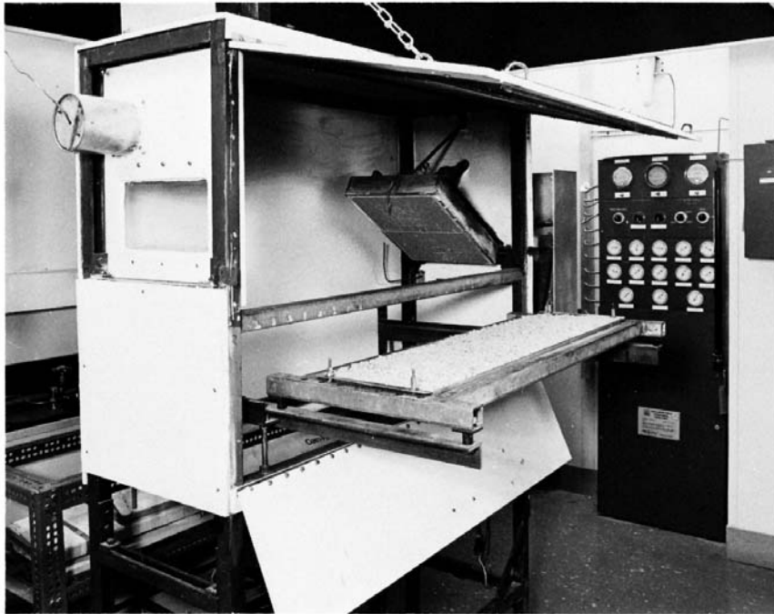
FIG. X1.1 Historic Photograph of Radiant Test Panel Chamber
