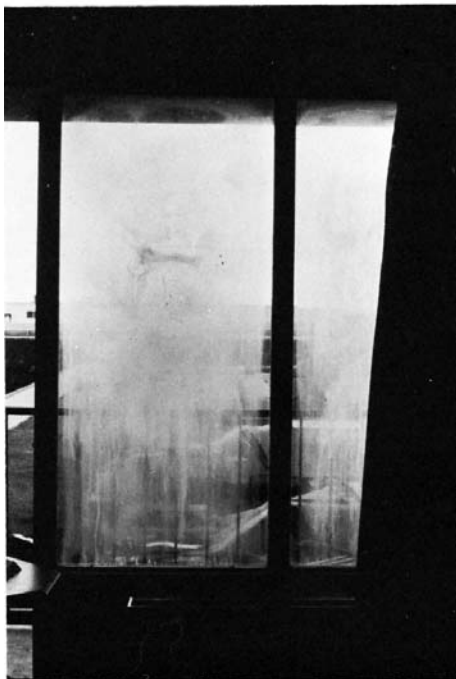
(b) Scummed and Stained Interior Glass Surface
