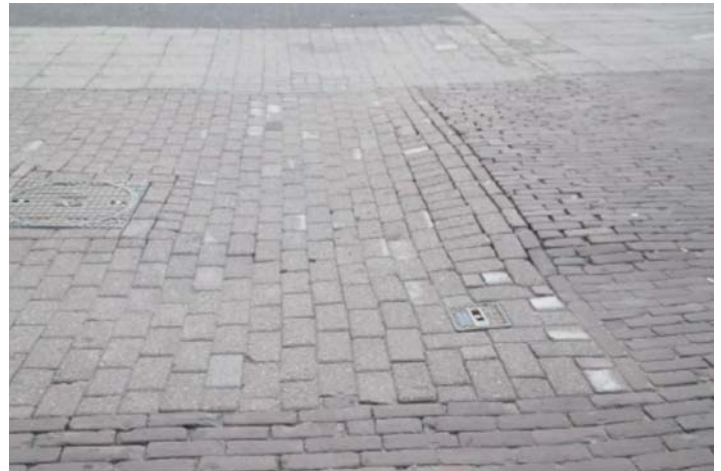
FIG. X1.17 Medium Severity Heave
