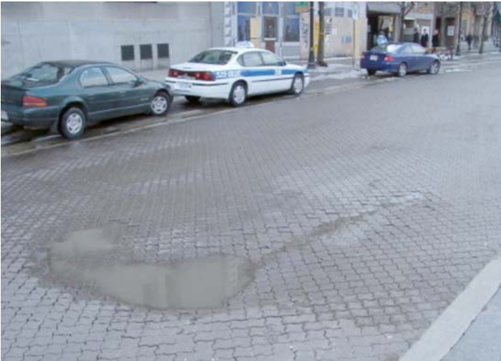
FIG. X1.6 High Severity Depression
