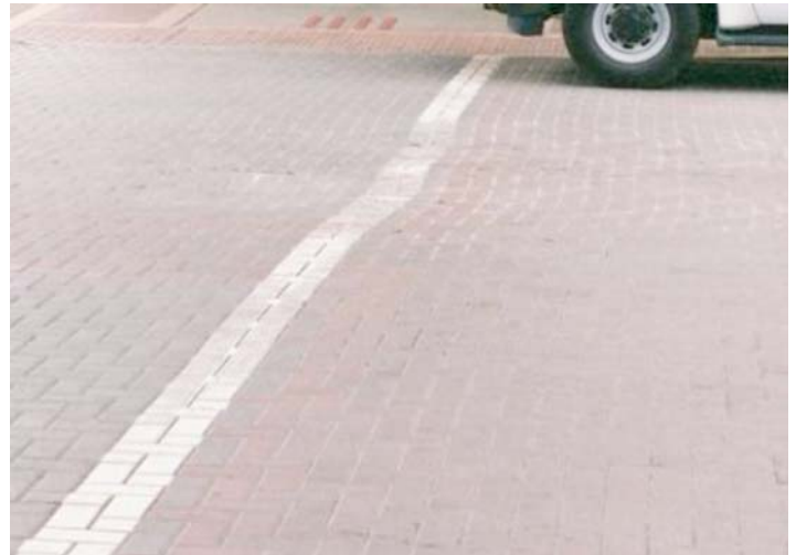
FIG. X1.5 Medium Severity Depression
