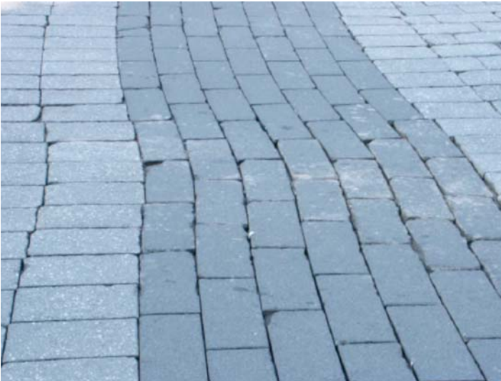
FIG. X1.21 High Severity Horizontal Creep
