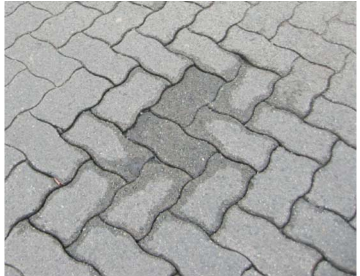
FIG. X1.10 Low Severity Excessive Joint Width (Approximately 1/4 in. (6 mm) wide and performing well)
