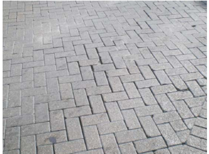
FIG. X1.19 Low Severity Horizontal Creep
