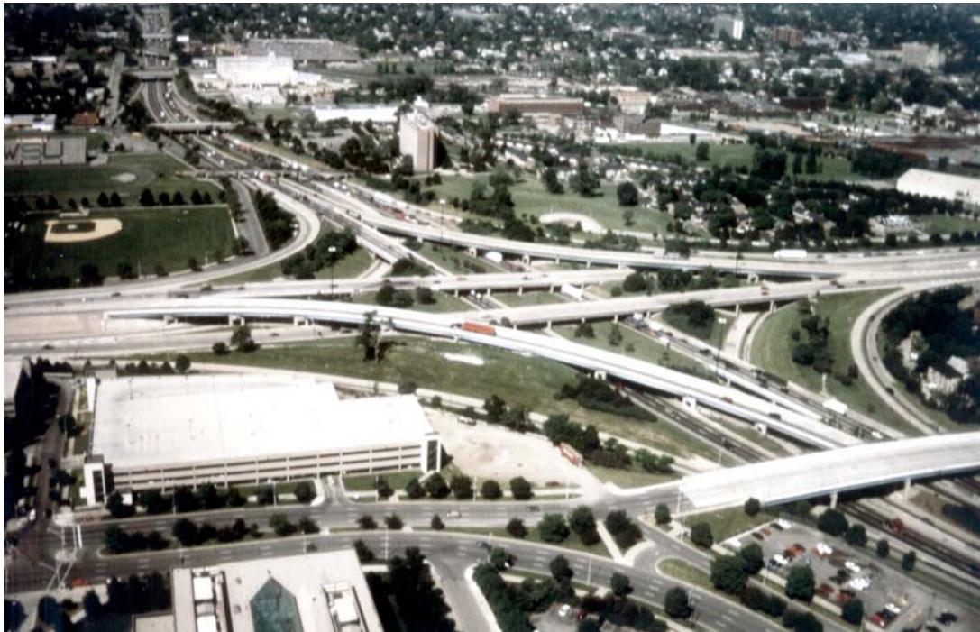
FIG. X2.1 Aerial View of I-94 Interchange
