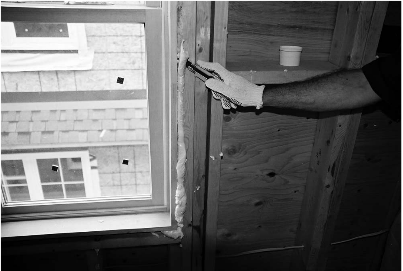
FIG. A1.5 Excess Type A Material Trimmed with a Sharp Knife
