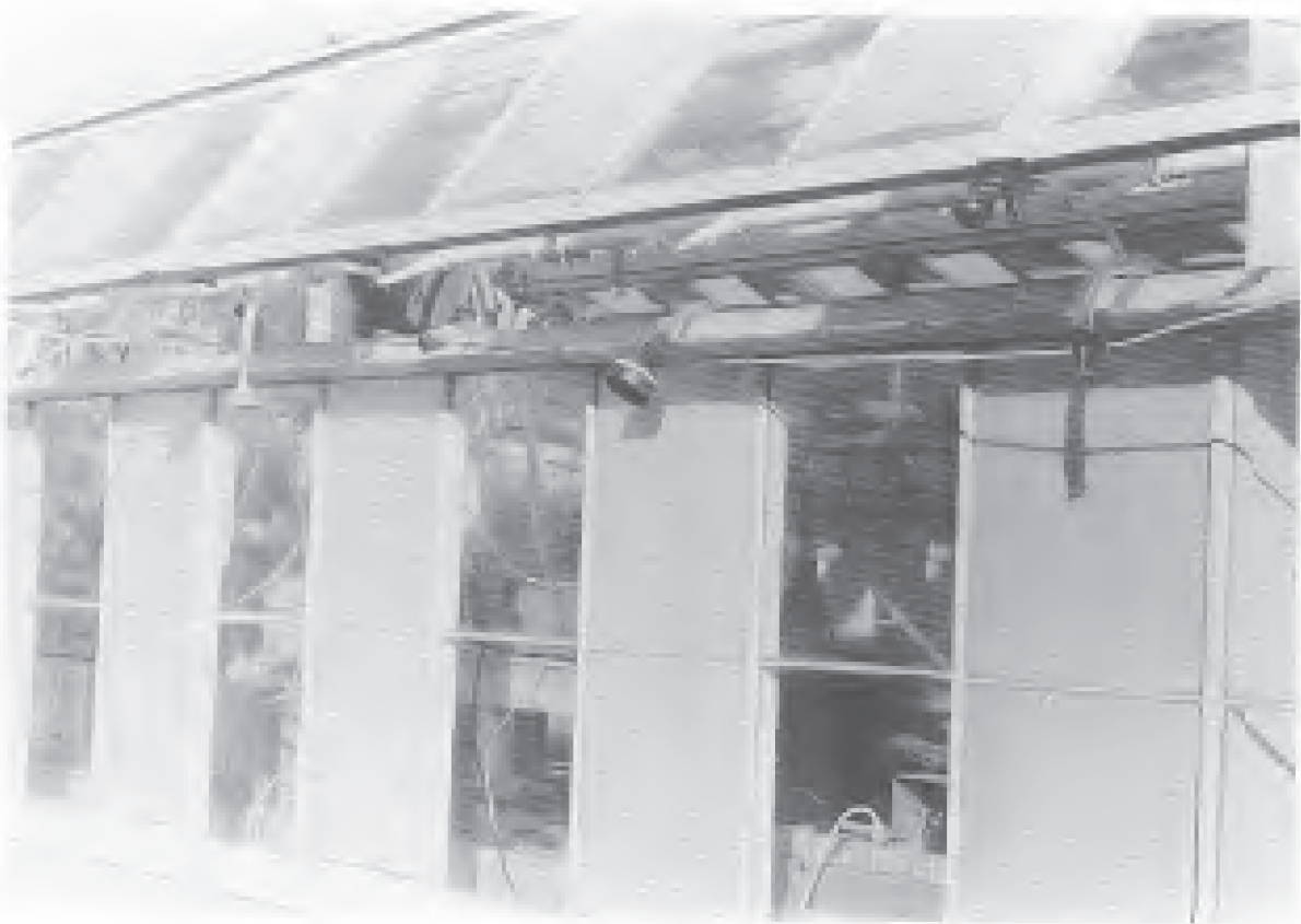
FIGURE 3. TAPE SAMPLER PROBE ARRANGEMENT AT THE BLOOMINGTON SITE
