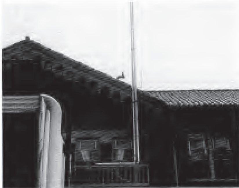
FIGURE 8. SULFUR DIOXIDE SAMPLING SYSTEM INTAKE LINE AT LOS ANGELES TEST SITE
