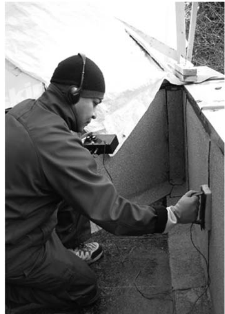
FIG. 6 Testing a Wall Seam with the Vertical Surface Unit
