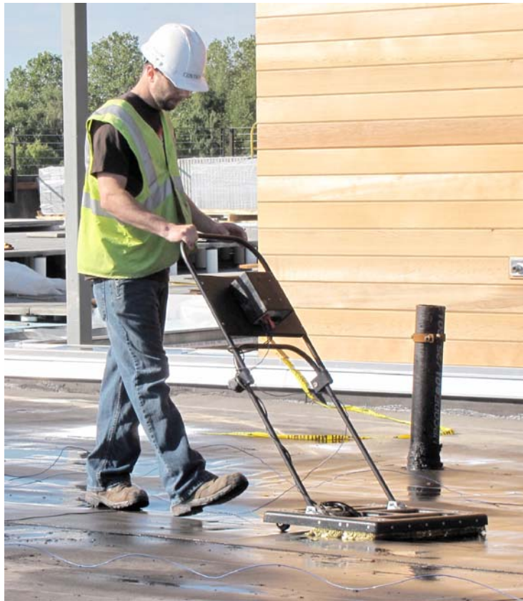
FIG. 2 Testing a Membrane with a Scanning Platform
