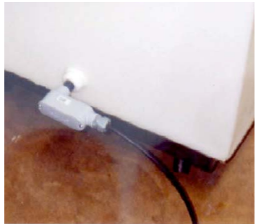
FIG. 6 Heater Conduit Boc Installed on Tank
