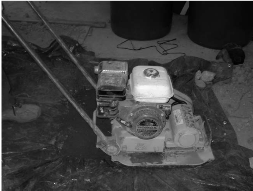
FIG. X1.3 Compaction of the Soil in the 2 ft by 2 ft Test Pit
