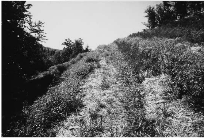
FIG. 4 Photograph of Live Fascines in the First Growing Season
