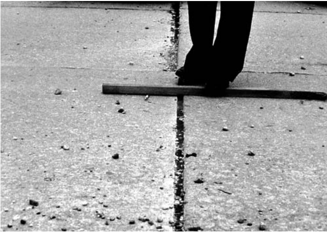
FIG. X2.13 Low-Severity Faulting
