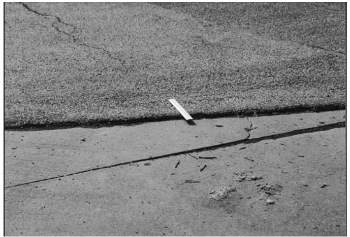
FIG. X1.45 Medium-Severity Shoving
