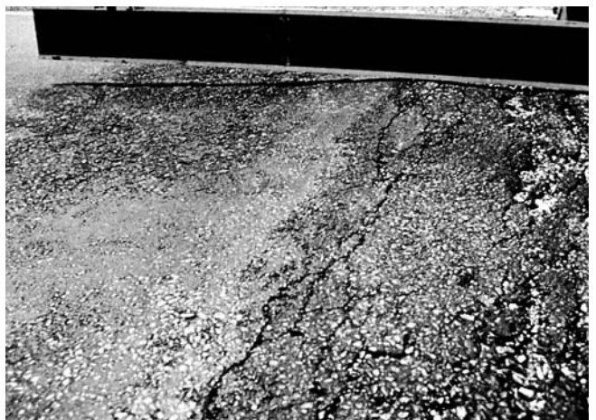
FIG. X1.12 High-Severity Bumps and Sags
