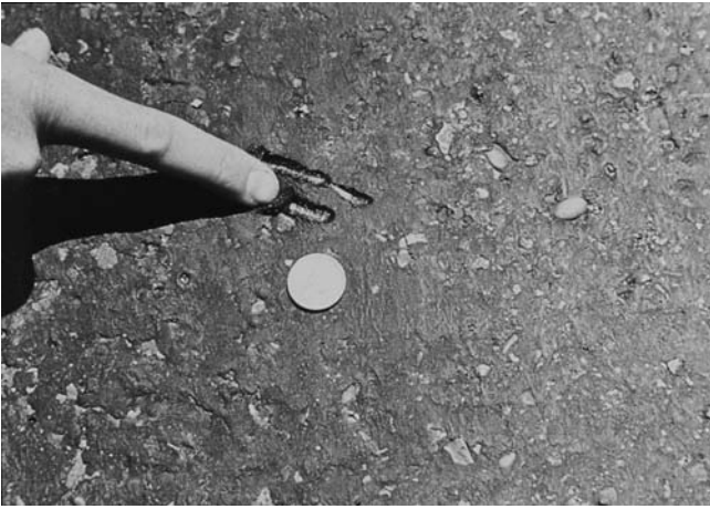
FIG. X1.5 Medium-Severity Bleeding
