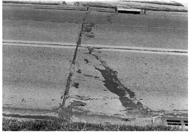
FIG. X2.36 Medium-Severity Punchout
