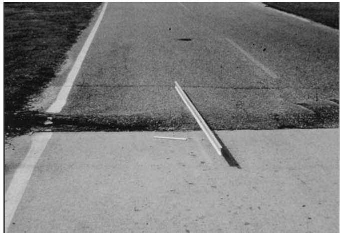
FIG. X1.46 High-Severity Shoving
