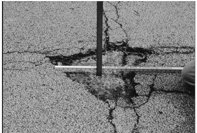
FIG. X1.36 Medium-Severity Pothole
