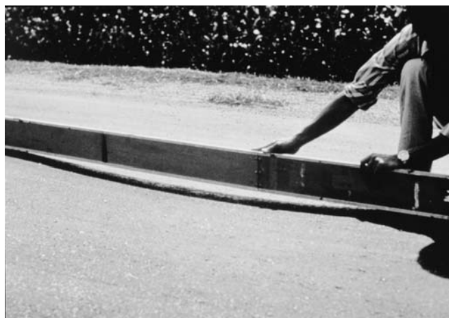
FIG. X1.17 Medium-Severity Depression
