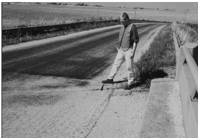
FIG. X1.44 Low-Severity Shoving
