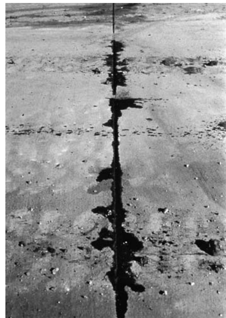
FIG. X2.33 Pumping
