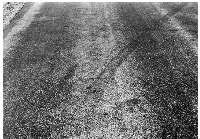
FIG. X1.4 Low-Severity Bleeding
