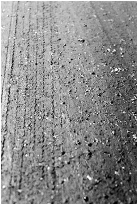
FIG. X1.6 High-Severity Bleeding
