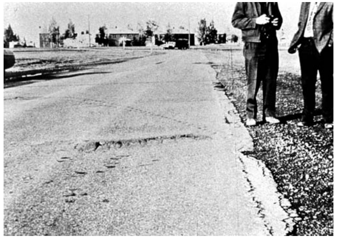
FIG. X1.11 Medium-Severity Bumps and Sags
