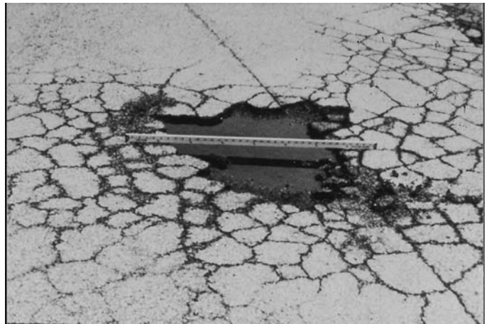
FIG. X1.37 High-Severity Pothole
