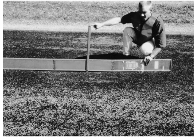
FIG. X1.16 Low-Severity Depression
