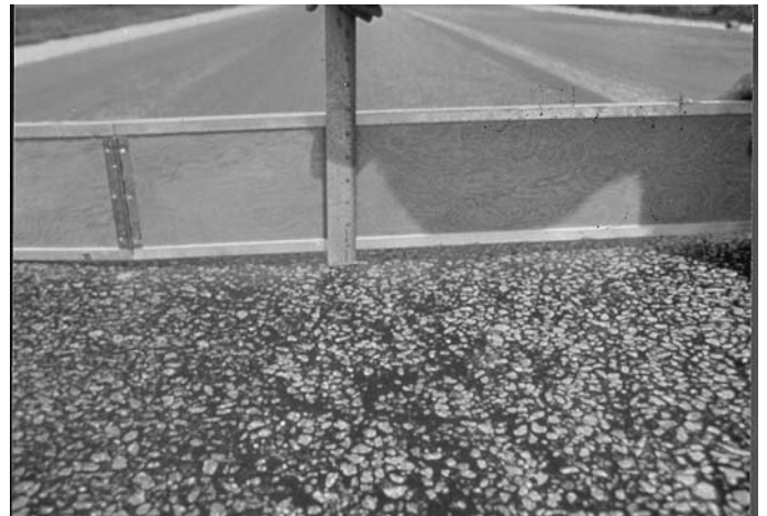
FIG. X1.42 Medium-Severity Rutting
