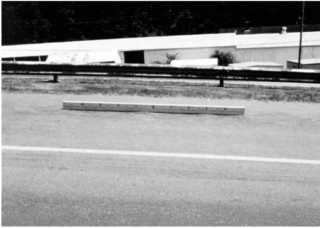
FIG. X1.14 Medium-Severity Corrugation
