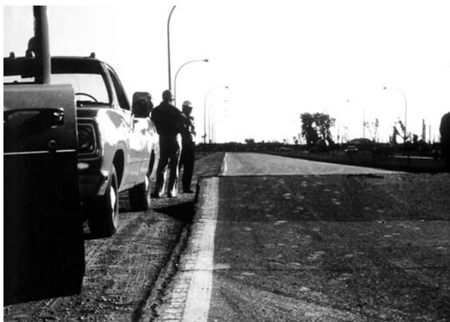
FIG. X2.3 High-Severity Blowup/Buckling
