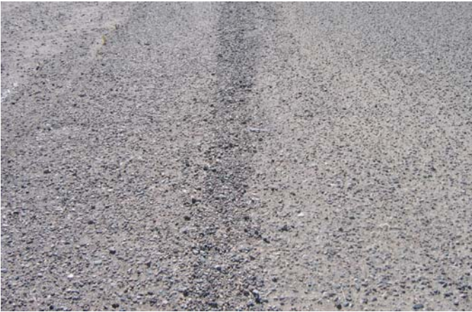
FIG. X1.52 High-Severity Raveling
