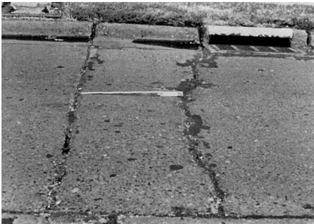
FIG. X2.35 Low-Severity Punchout
