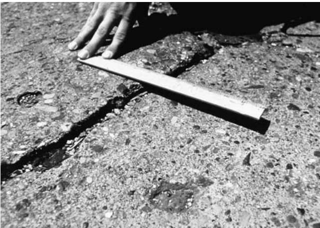
FIG. X2.14 Medium-Severity Faulting
