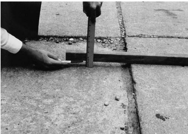
FIG. X2.15 High-Severity Faulting
