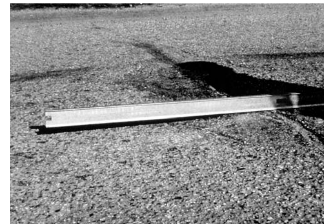
FIG. X1.10 Low-Severity Bumps and Sags
