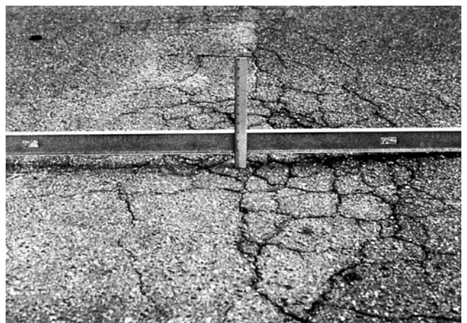
FIG. X1.18 High-Severity Depression
