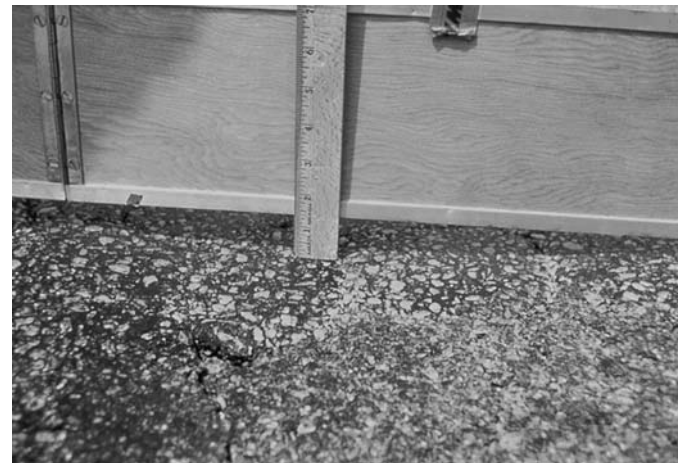
FIG. X1.43 High-Severity Rutting
