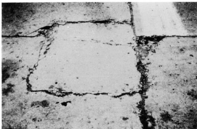
FIG. X2.37 High-Severity Patch
