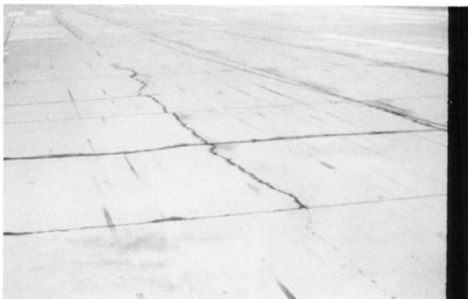
FIG. X2.53 Low-Severity Intersecting Cracks
