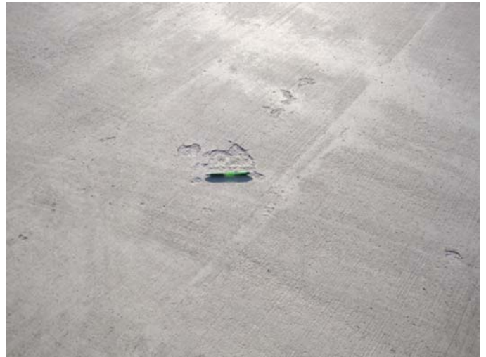
FIG. X2.44 Low-Severity Scaling
