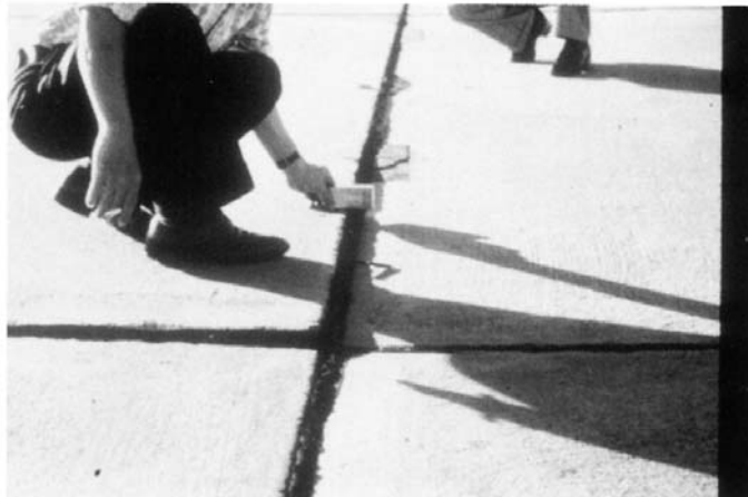
FIG. X2.52 High-Severity Settlement
