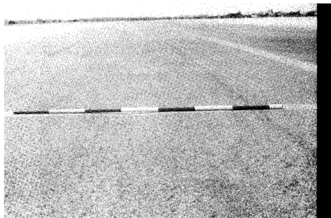
FIG. X1.66 Low-Severity Rutting
