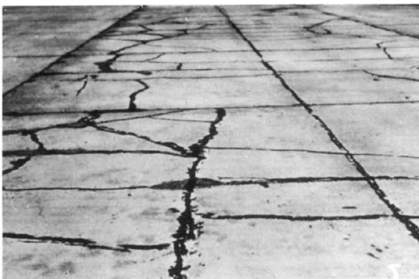
FIG. X2.57 Shattered Slab
