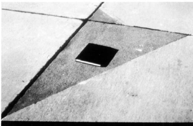
FIG. X2.33 Low-Severity Patch
