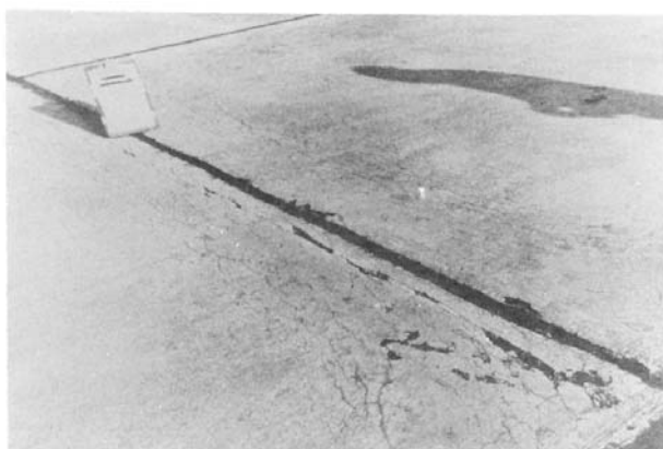
FIG. X2.22 High-Severity "D" Cracking
