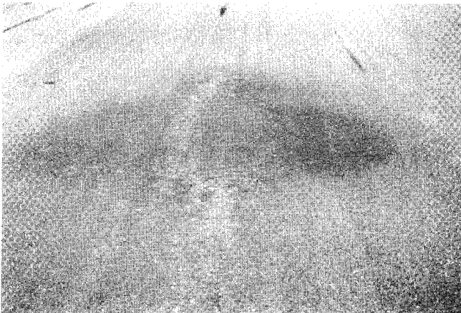
FIG. X1.24 Low-Severity Depression
