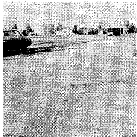
FIG. X1.77 High-Severity Swell
