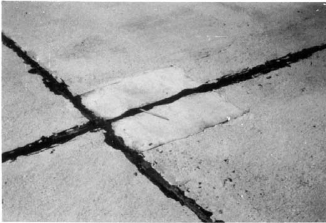
FIG. X2.28 Low-Severity Small Patch
