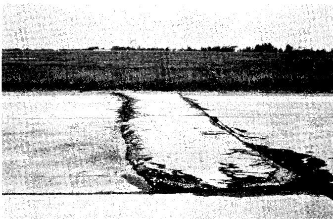
FIG. X2.2 Medium-Severity Blowup
