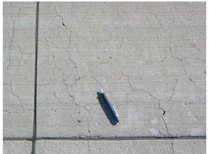
FIG. X2.75 Medium-Severity ASR
