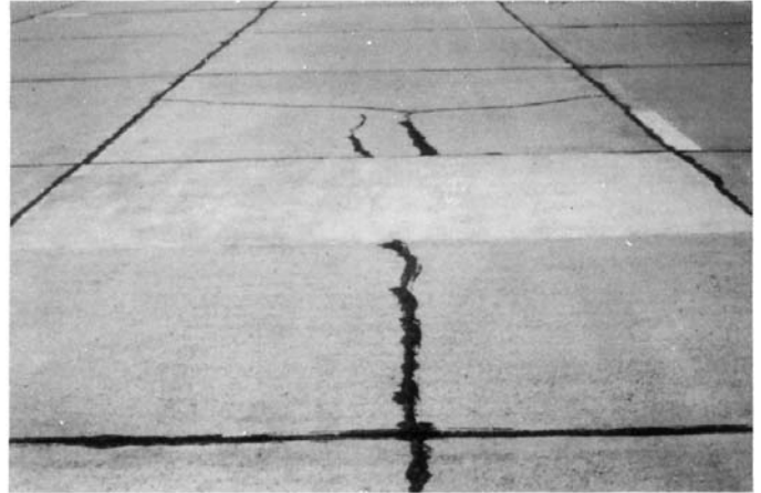
FIG. X2.34 Low-Severity Patch
