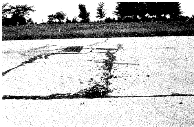
NOTE 1—This would only be considered low severity if the shattering in the foreground was the only part existing and the foreign material removed.
