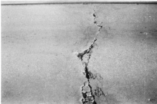
FIG. X2.15 High-Severity Crack
