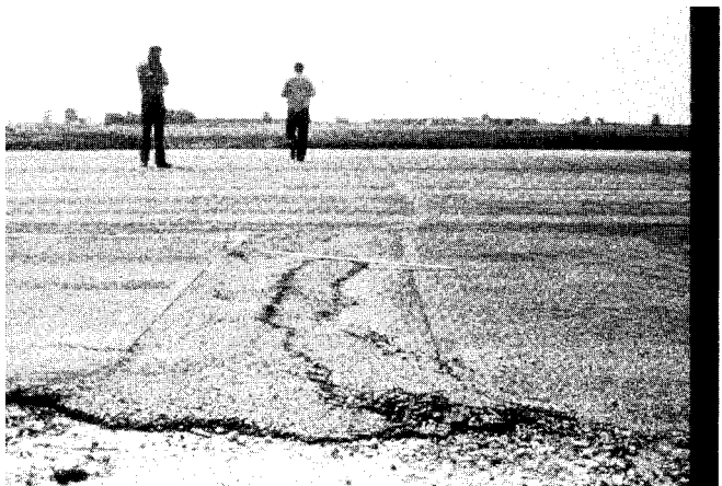
FIG. X1.52 High-Severity Patch
