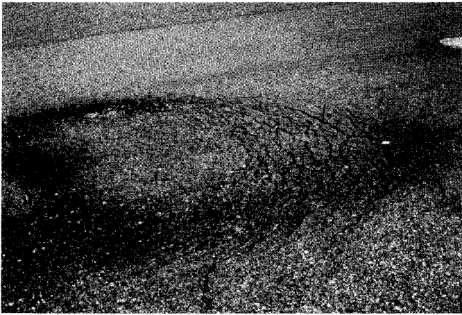
FIG. X1.73 Slippage Cracking
