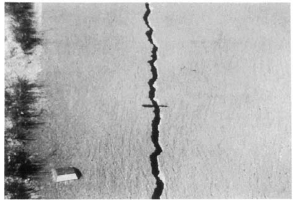
FIG. X2.17 High-Severity Crack
