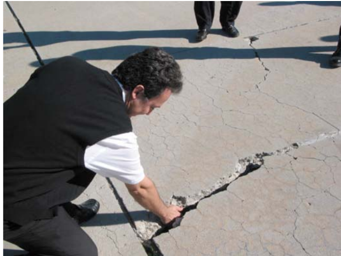
FIG. X2.76 High-Severity ASR
