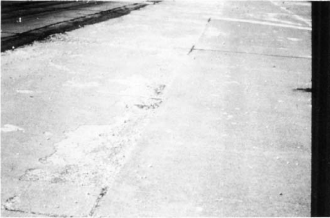
FIG. X2.46 High-Severity Scaling
