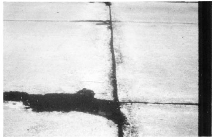
FIG. X2.45 Medium-Severity Scaling
