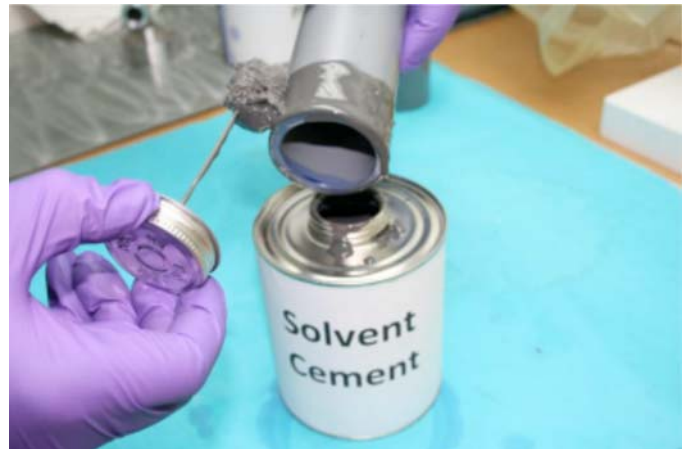
FIG. 13 Apply a full, even layer of solvent cement to the pipe end beyond the mark delineating the depth of the fitting socket.
