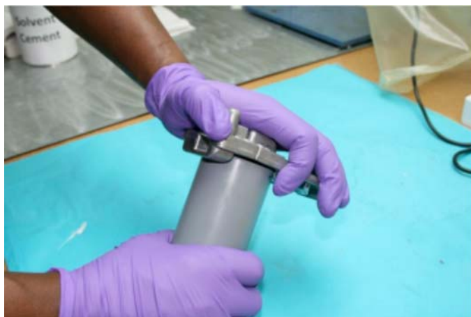
FIG. 7 Deburr and Chamfer the Pipe End
