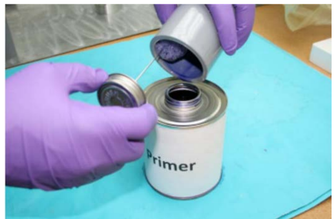
FIG. 11 Apply primer to the fitting socket.
