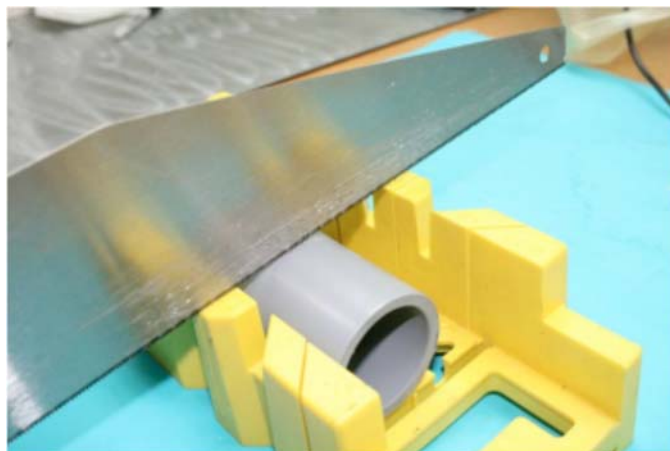
FIG. 5 Cut the pipe straight at a 90° angle.
