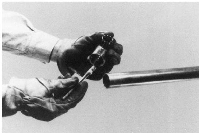
FIG. 11 Fluxing: Fitting
